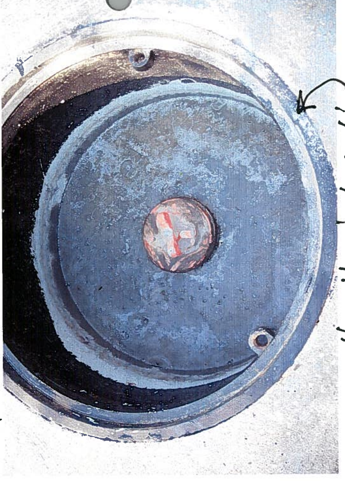
Material used to seal concrete, in vaults
