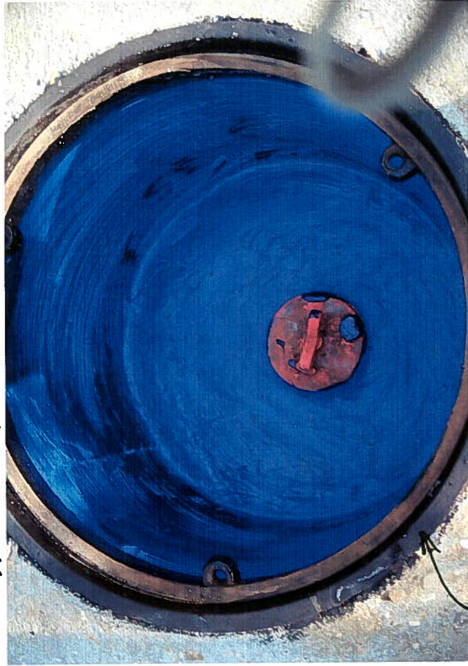
Well vaults after sealant applied
