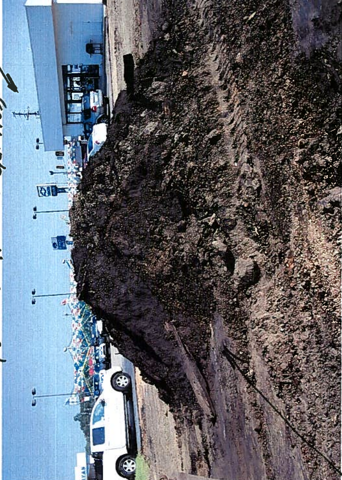
Soil sample collected from soil pile to determine disposal options
