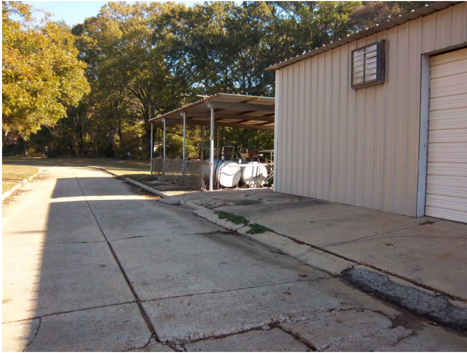
Photograph 15: View of the northwest corner of the vehicle maintenance shop showing the adjacent metal canopy and the diesel and unleaded gasoline ASTs where vehicles are fueled.
