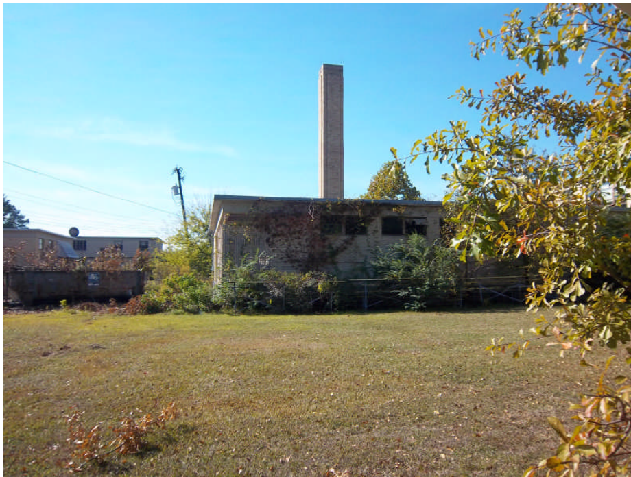
Photograph 11: View of the cafeteria and boiler stack on the subject property.
