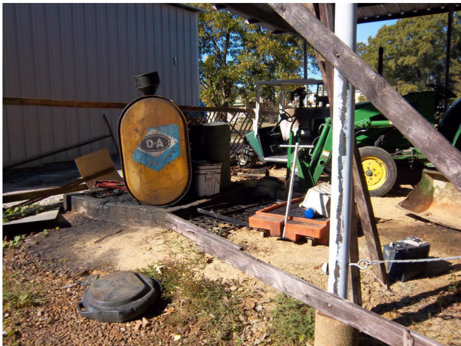
Photograph 16: View of the used oil AST showing soil staining. Note the overturned oil drain pan on the ground surface, the portable oil drain catch pan, and the damaged automotive battery stored on the ground surface.
