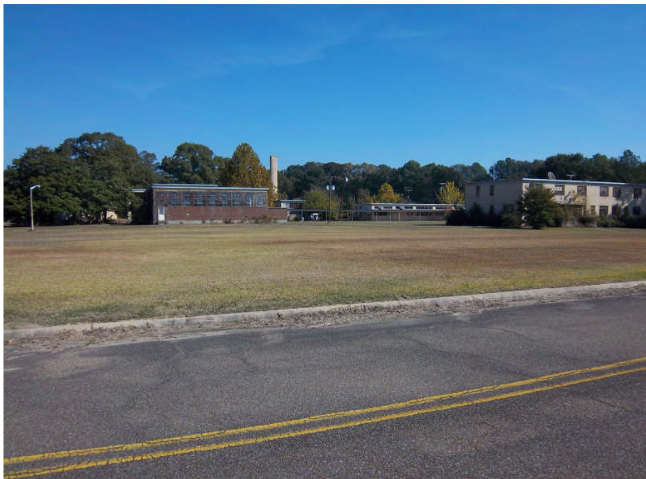
Photograph 8: General view of the subject property from the southern boundary looking north. From left to right is the indoor swimming pool, the cafeteria boiler stack, and the administration building.
