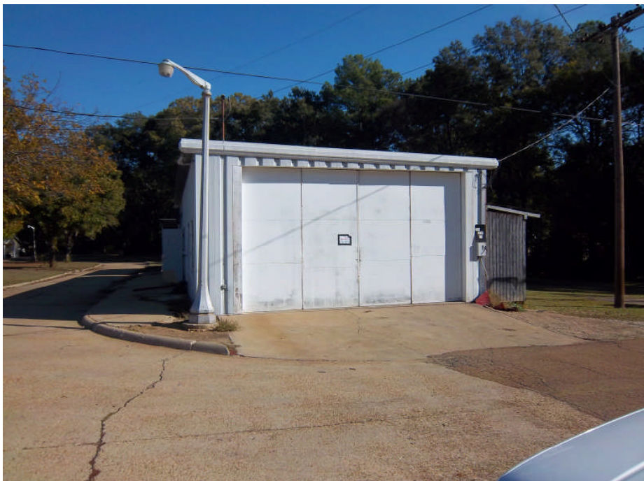
Photograph 14: View of the south side of the vehicle maintenance shop looking north.
