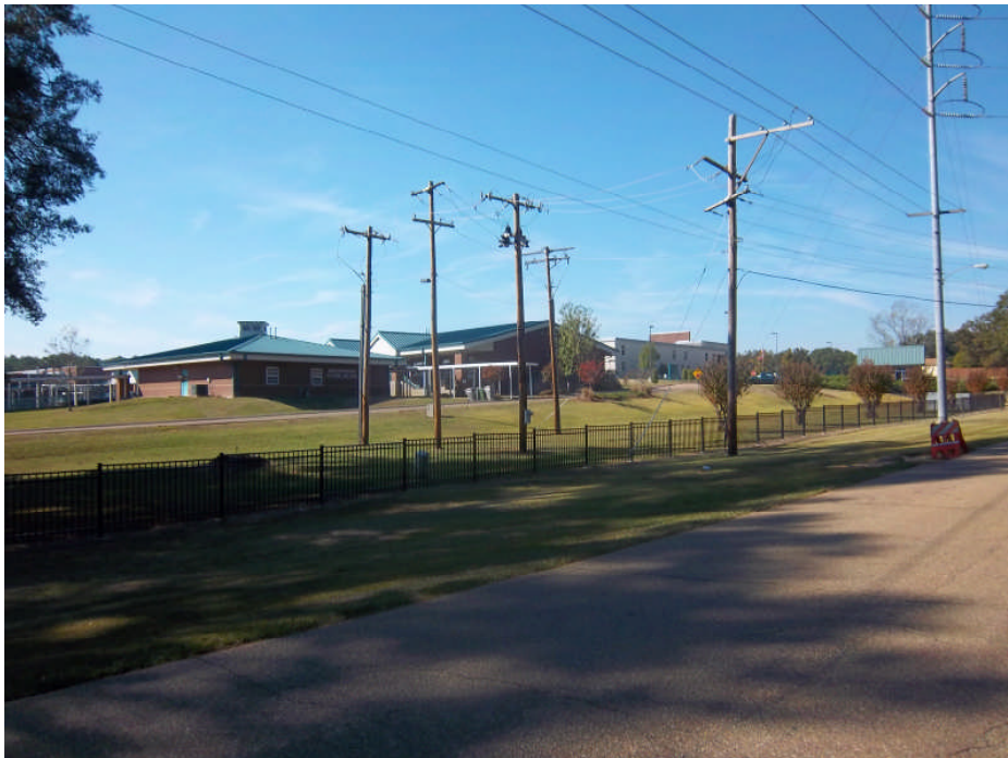
Photograph 21: View looking southwest at the adjacent Mississippi School for the Blind and Deaf to the south of the subject property.
