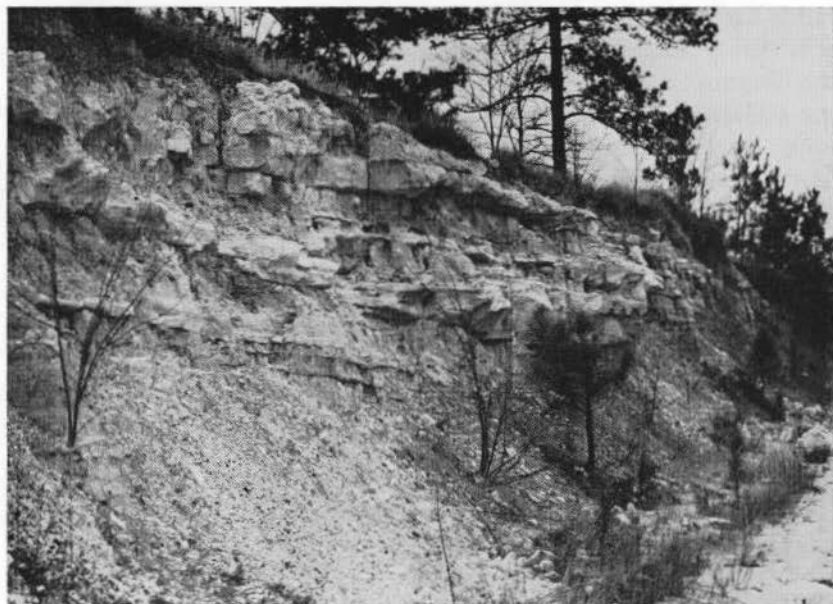
Figure 28.—Interbedded Catahoula sandstones and clayey silts exposed in roadcut on State Highway 27 near Bear Creek Church in NW.¼, Sec.32, T.3N., R.3W. Perry Nations photo. March 5, 1965.
