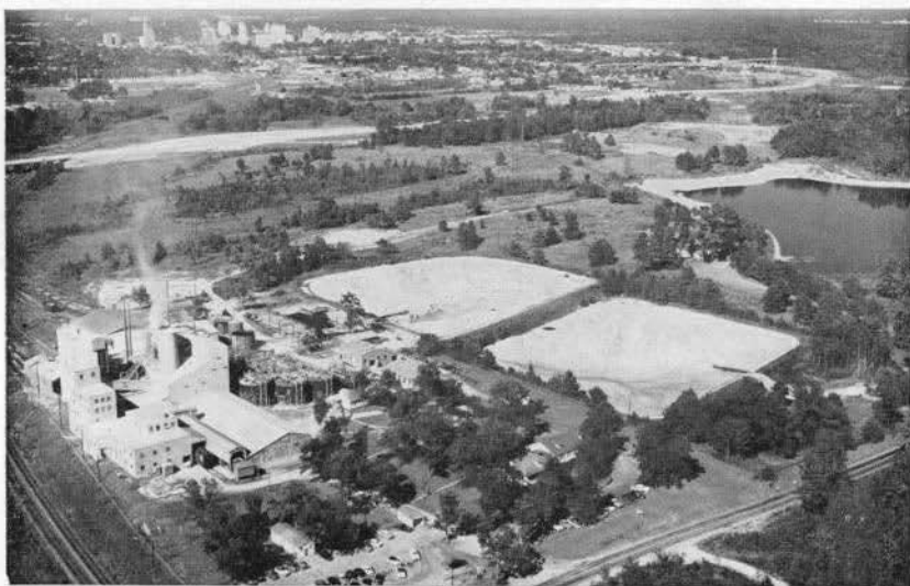
Figure 8.—Filtrol Corporation's bentonite activation plant at Jackson. Looking northeast. (M.G.S. Bull. 86, Fig. 21). Photo by Manley, Tucson.
