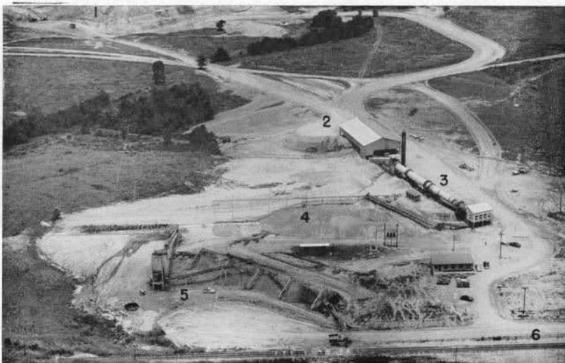
Figure 6.—Lightweight Aggregate Division plant of Jackson Ready-Mix Concrete at Cynthia: (1) pits opened in the Yazoo clay, (2) clay dry shed, (3) rotary kiln, (4) cinder storage area, (5) grinding, screening and storage of graded aggregates, and (6) rail or truck shipping facilities. (M.G.S. Bull. 86, Fig. 24).—Frank Noone photo, July 2, 1958.
