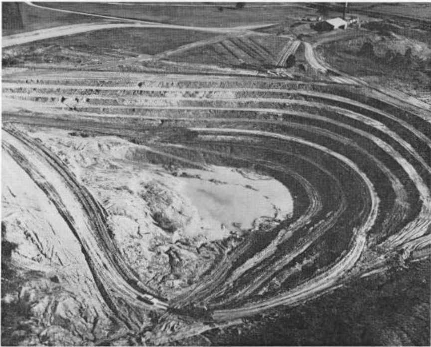
Figure 7. Open-cut pit of the Lightweight Aggregate Division, Jackson Ready-Mix Concrete (NE.¼, NW.¼, Sec.36, T.7N., R.1W.). The mine is over 60 feet deep. Note the several tiered benches from which the clay is worked.—Bob Hand photo.
