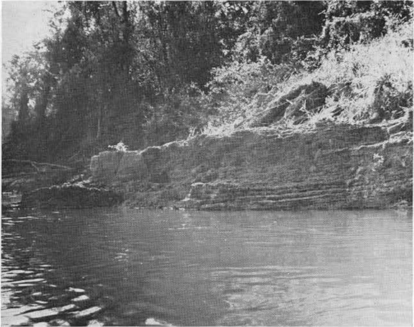
Figure 34.—Dip in alluvium (slump) in west bank of Pearl River in Sec.36, T.6N., R.1E. Perry Nations photo. September 22, 1964.
