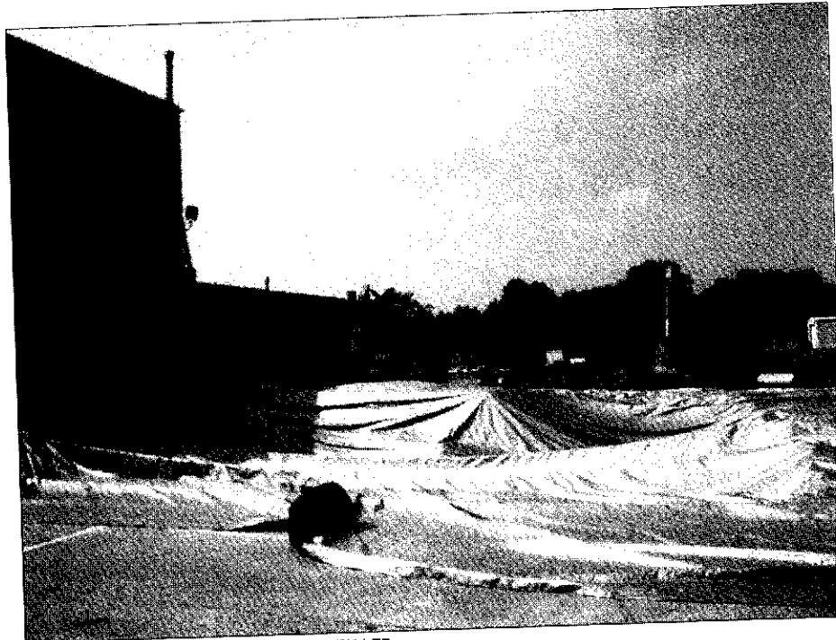
PHOTO 9 STORMWATER DETERRENT SYSTEM INSTALLED
