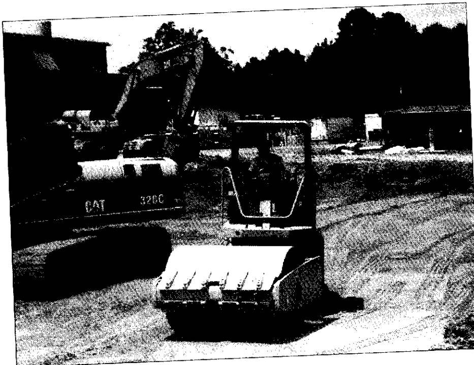
PHOTO 14 COMPACTION OF FILL MATERIAL
