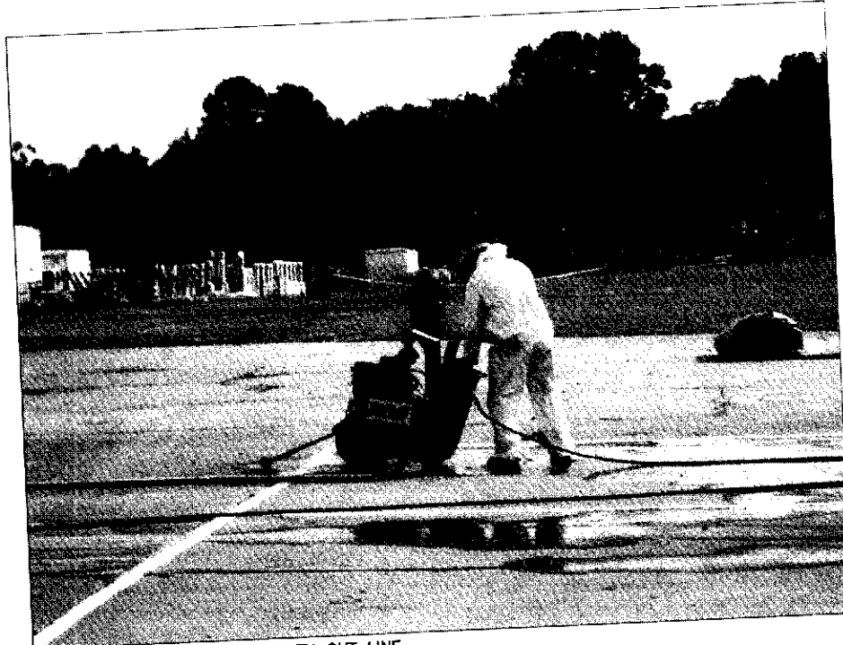
PHOTO 5 CONCRETE CUTTING ALONG SOUTH CUT LINE
