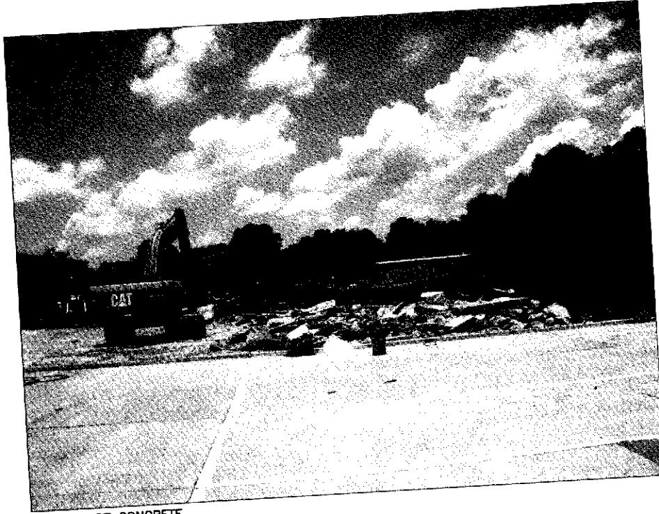
PHOTO 7 REMOVAL OF CONCRETE
