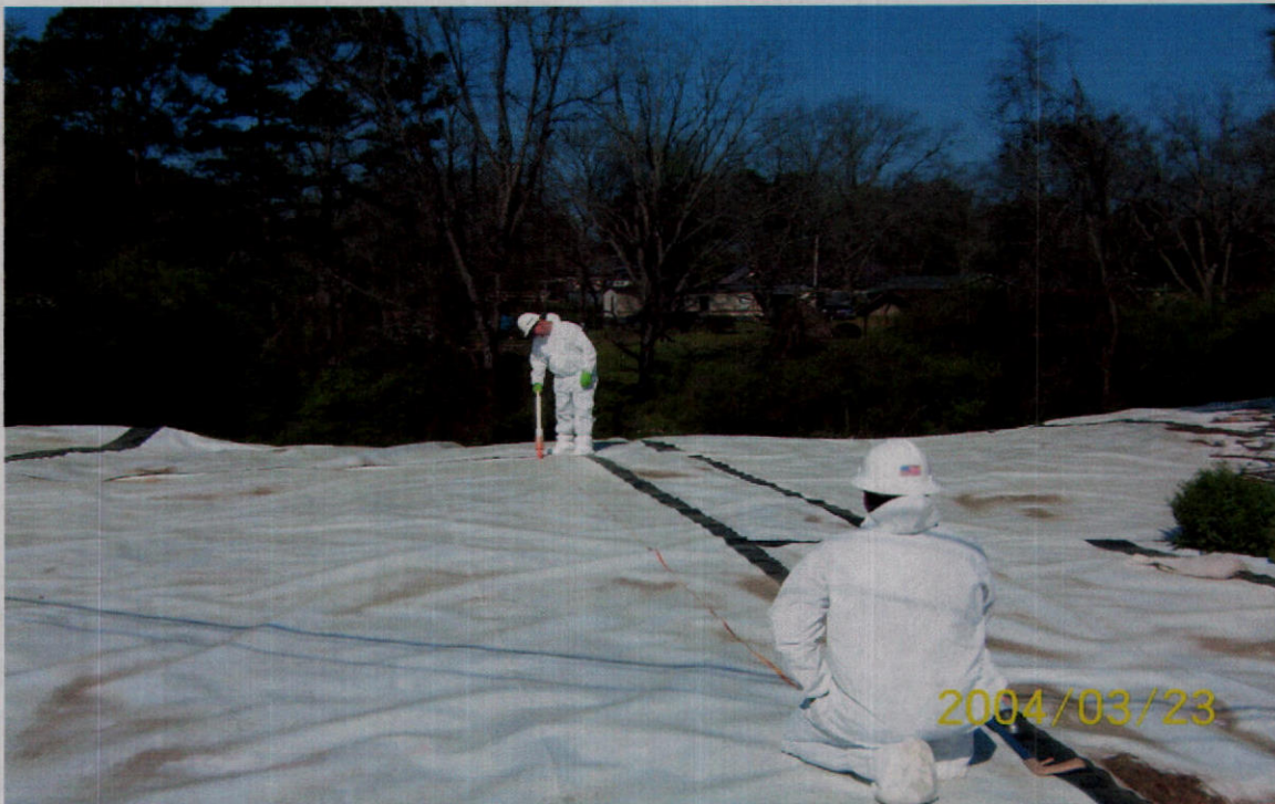
PHOTO 3 – Schnabel Engineering personnel laying out the X-Y survey grid for the geophysical study. Photo was taken looking east to west on the 114 Brent Street MSL property.
