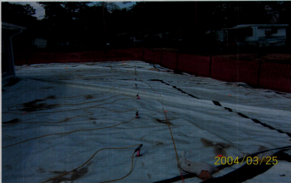
PHOTO 5 – Linear electrode array for the resistivity study portion of the geophysical survey. Photo was taken from the driveway to the house looking south to north.
