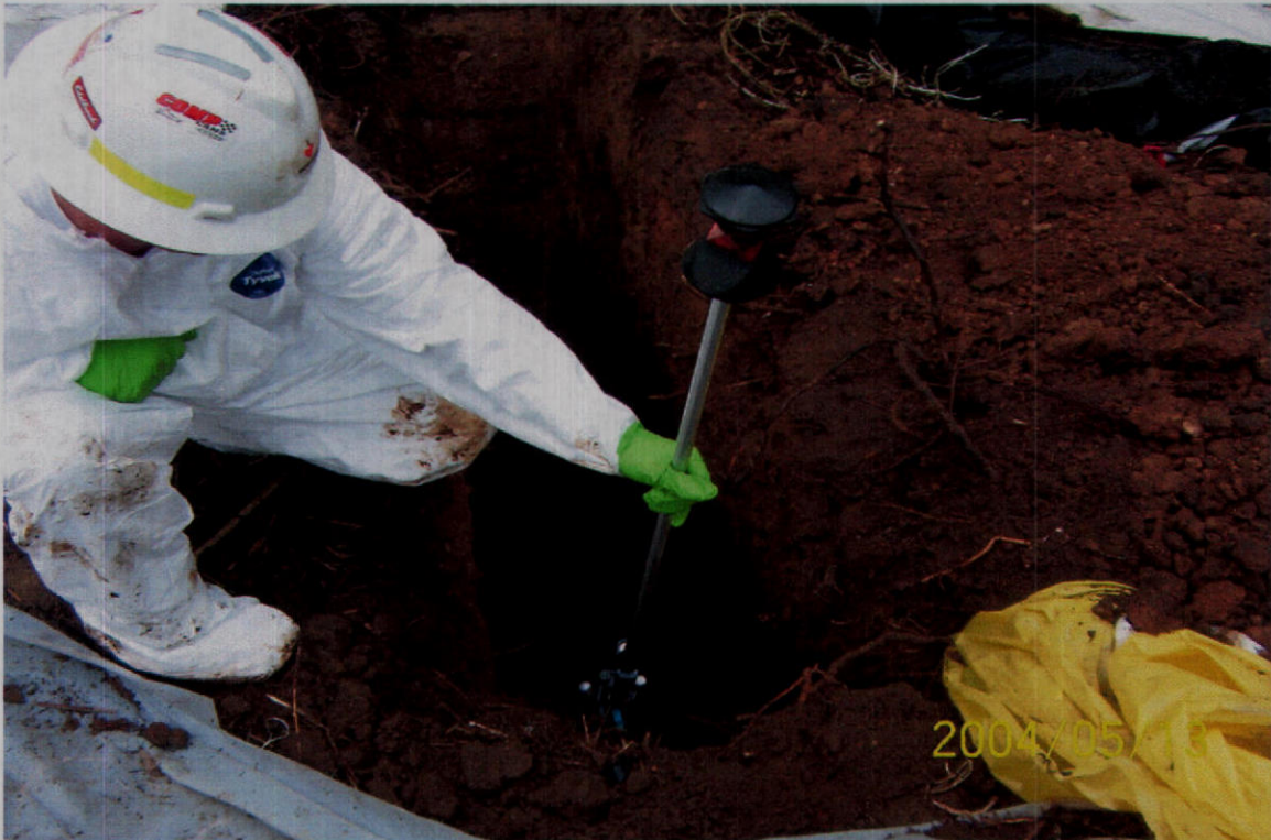
PHOTO 16 – A view of the surveyor gathering sample point coordinate data during installation of Test Pit #5. Test Pit #5 was located on the southeastern slope of the fill area.
