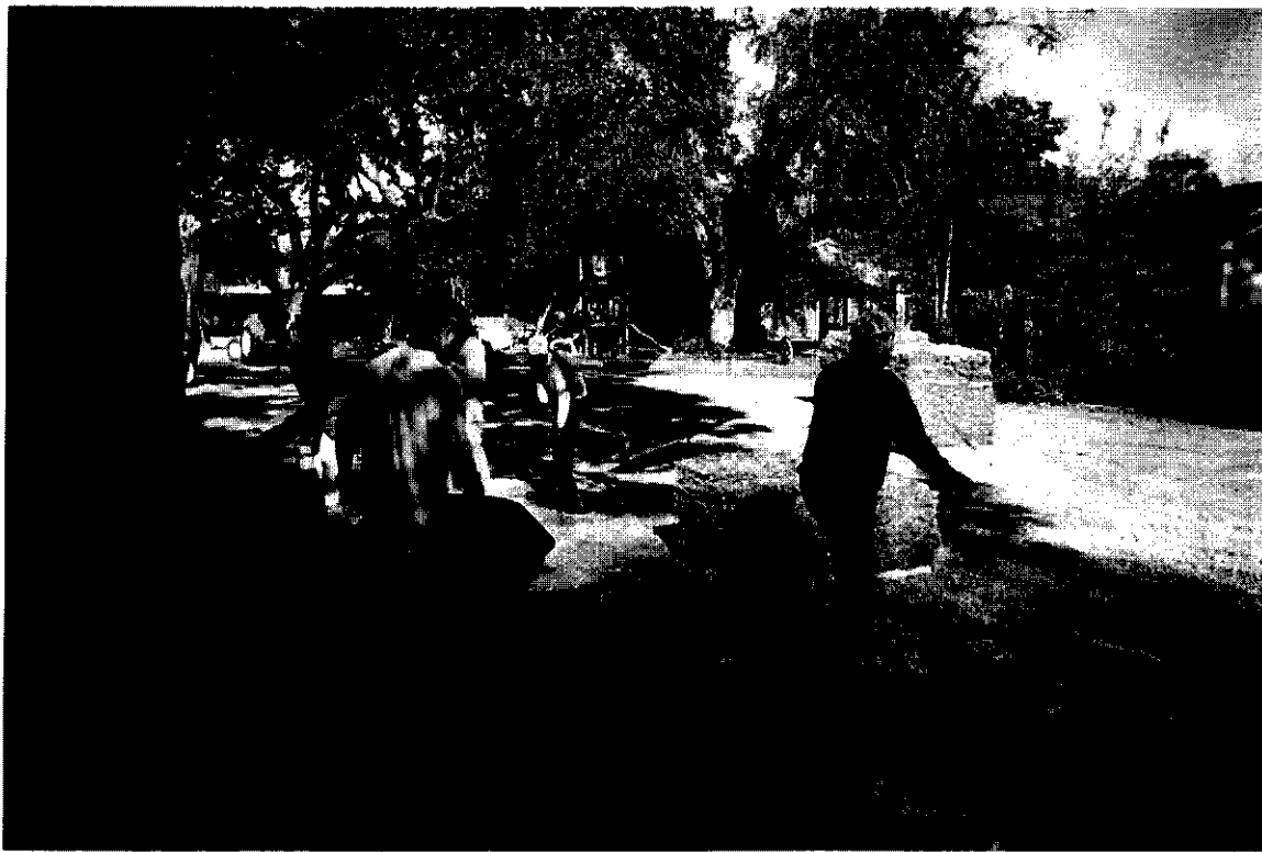
Dabney/Smith site looking north toward the residence showing installation of new sod on the Medical Center property and the adjacent Dabney/ Smith property.
