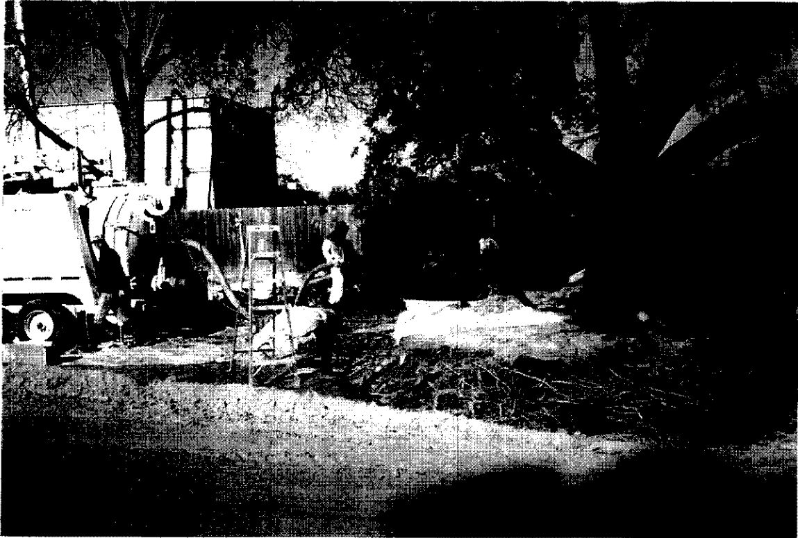
Dabney/Smith site looking north toward the KEC plant showing the cleaning of live oak tree roots using an Air Shovel™ to hydraulically remove soil without damaging the roots.
