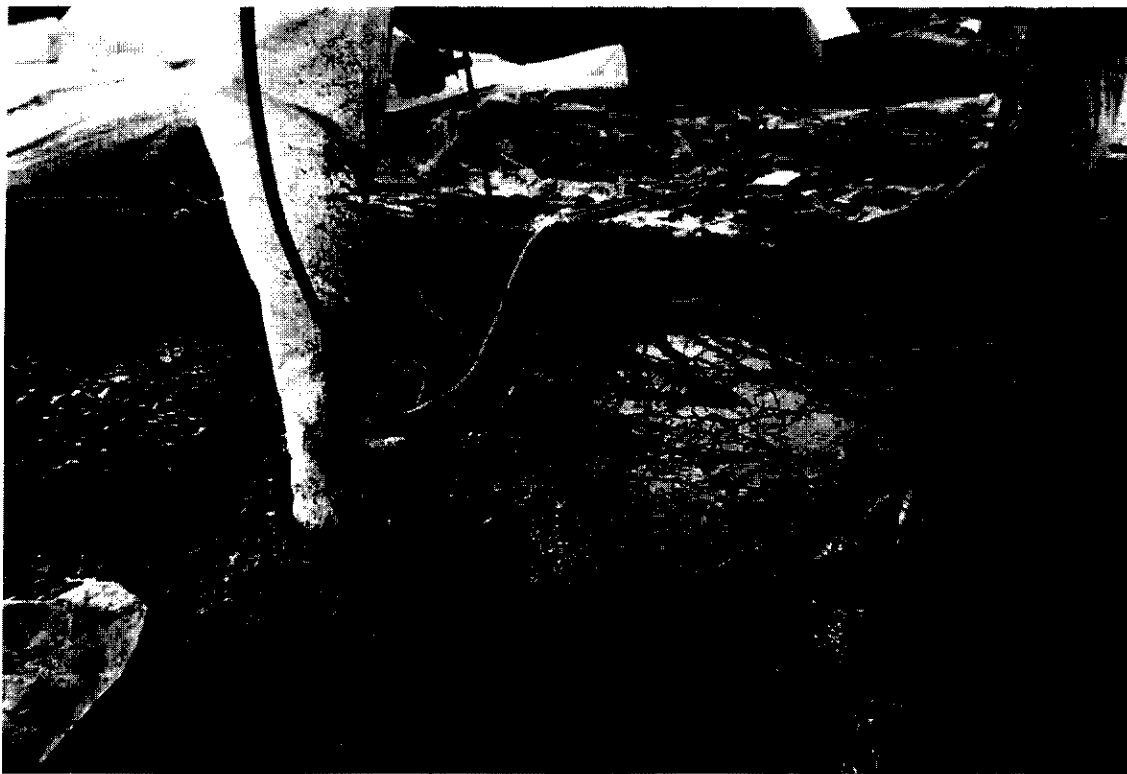
Dabney/Smith site showing a detail of soil removal using an Air Shovel™.
