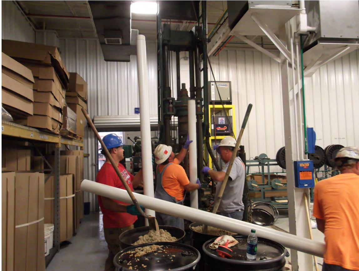
Installation of Deep Extraction Well
