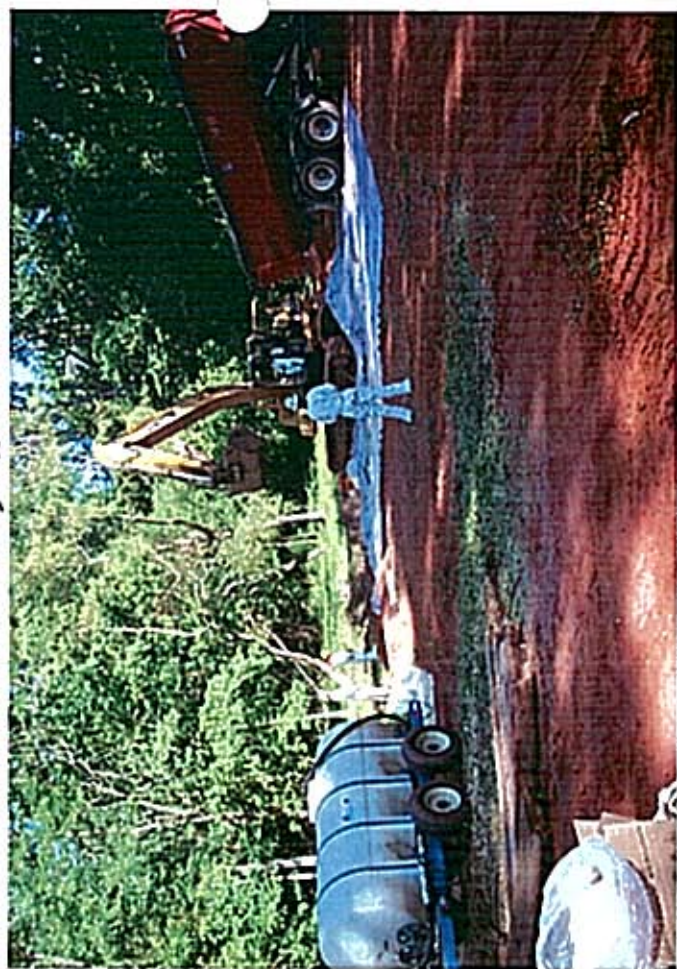
↳ LOADING EXCAVATED MATERIAL
