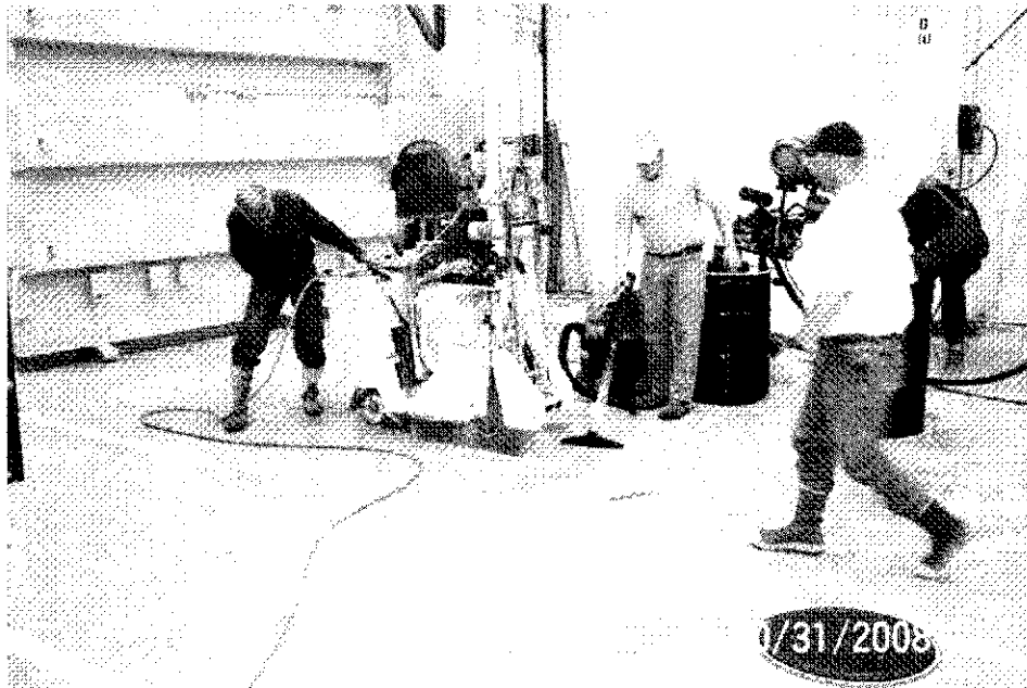
PHOTO 1 SAW-CUTTING CONCRETE AND RECOVERING RUN-OFF WATER.
