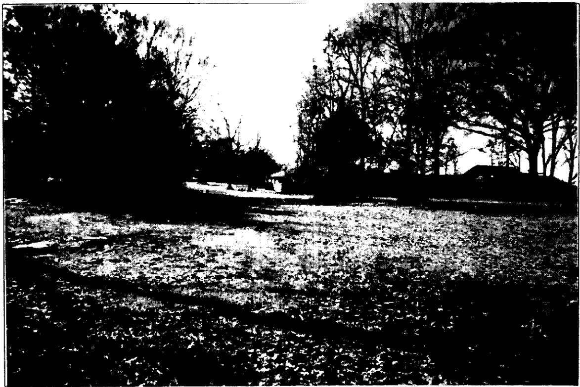
Completed project between Florence St. and Scooba St. (facing upstream)
