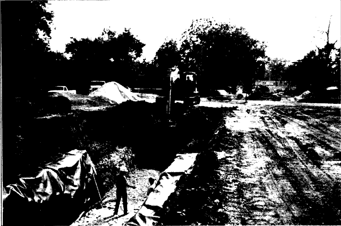
Trench excavation upstream of MLK Ave. (facing upstream)
