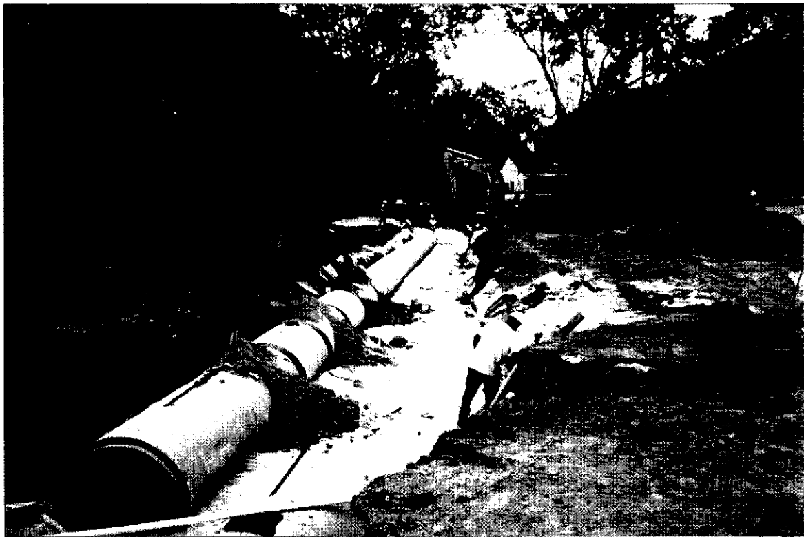
Culvert installation between Harrell St. and Florence St. (facing upstream)
