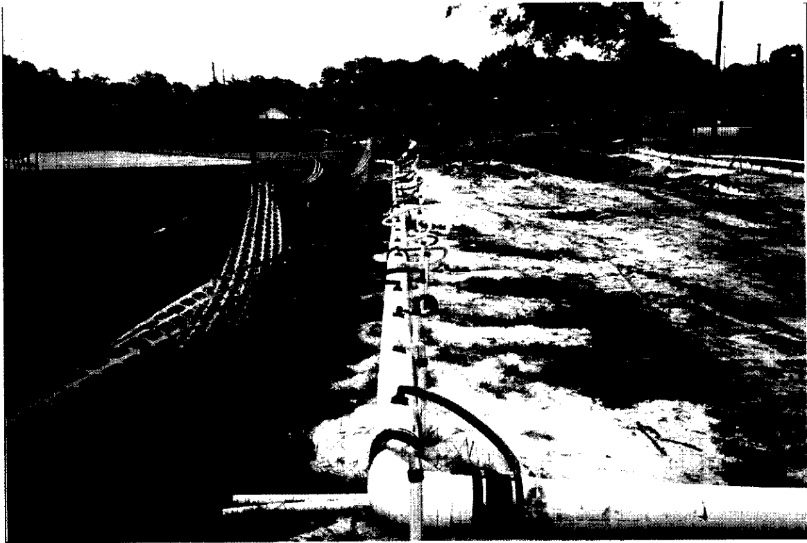
Shallow dewatering system adjacent to Francis St. Apts. (facing downstream)
