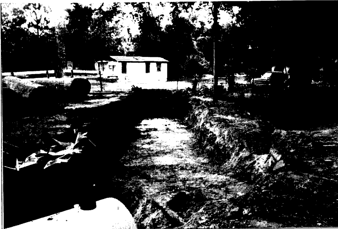
Trench excavation crossing Francis St. (facing upstream)
