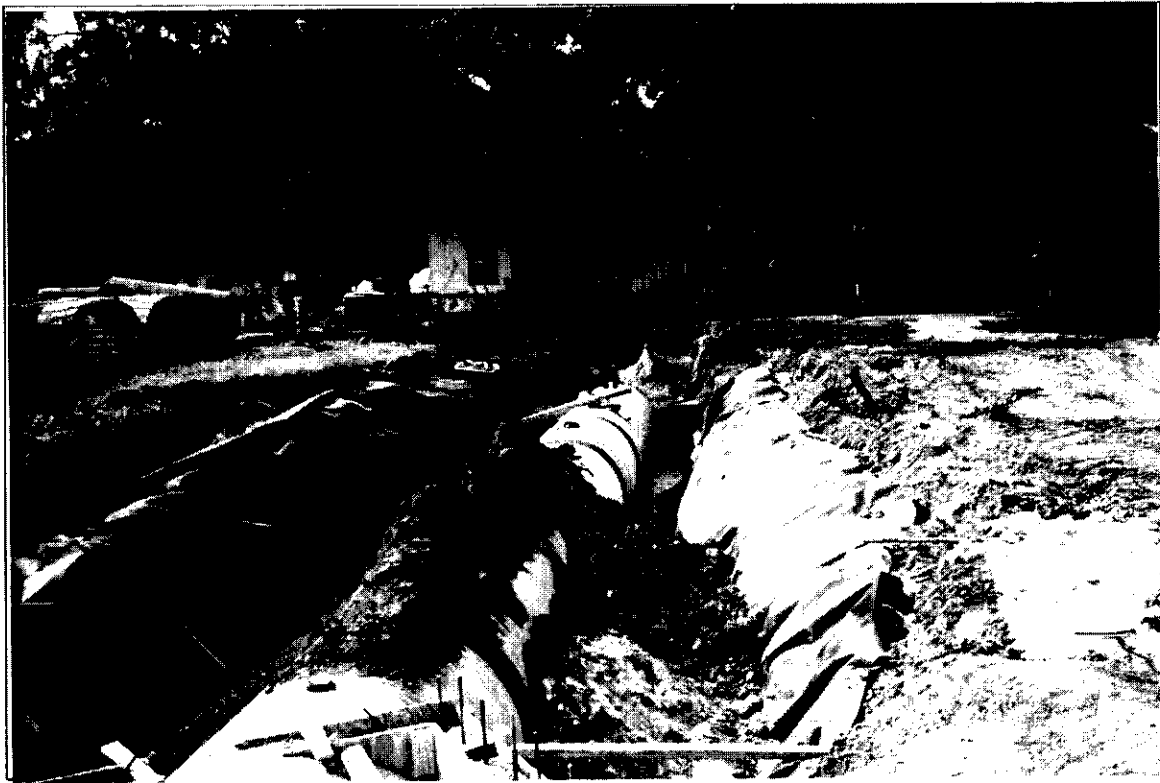
Culvert installation downstream of Francis St. (facing upstream)
