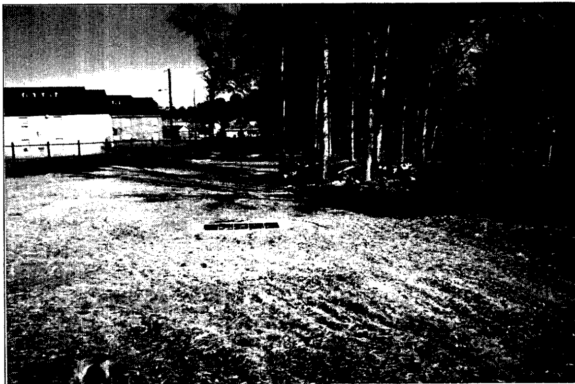
Completed project upstream of Francis St. Apts. (facing downstream)
