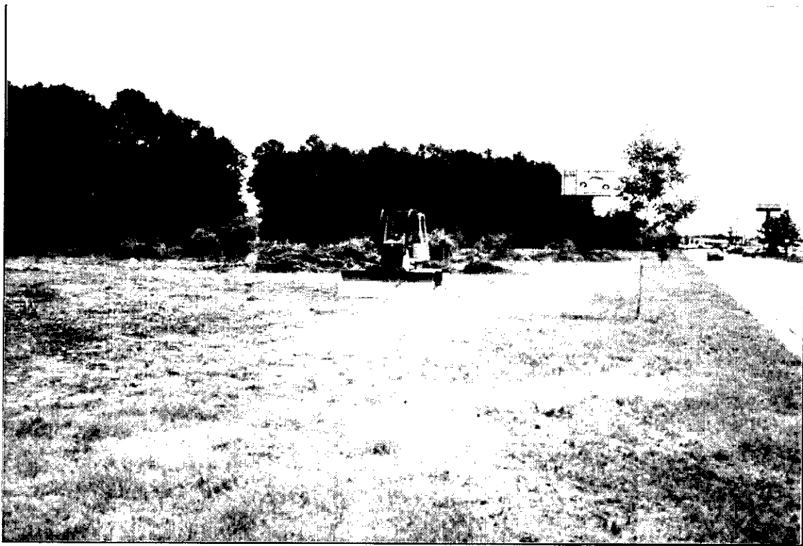
Gordon's Creek Fill Area during clearing and grubbing
