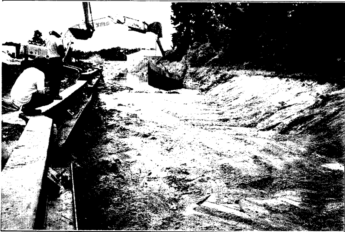
Removal of dam at upstream end of Gordon's Creek sediment removal area
