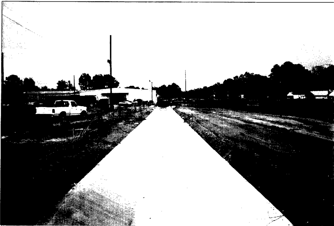
Completed concrete-lined ditch
