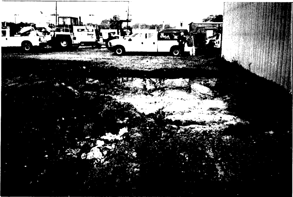
Removal of structurally incompetent material beneath base failures in former Process Area
