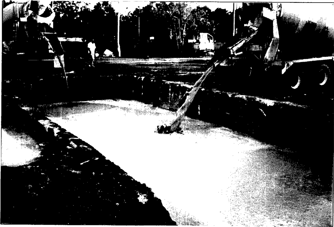
Filling concrete sump with flowable fill
