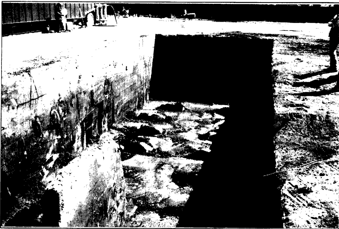
Cleaned out sump with concrete saddles at base
