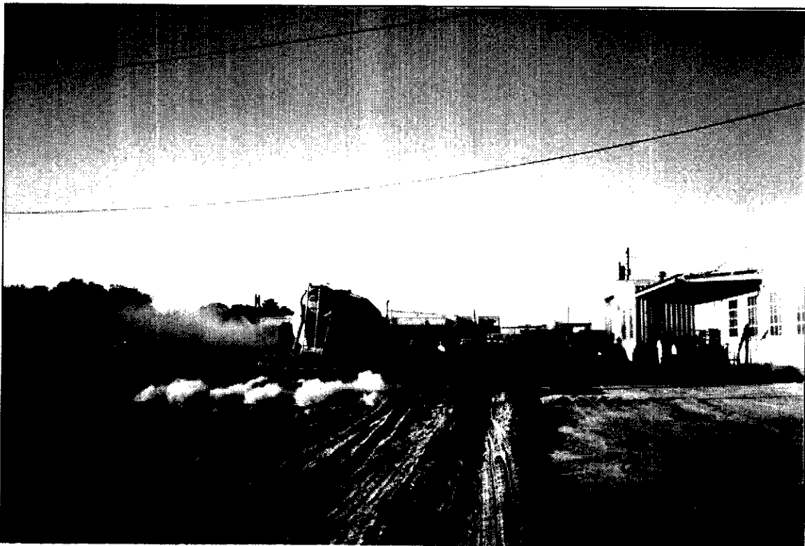
Application and mixing of stabilizing agent (soil cement)
