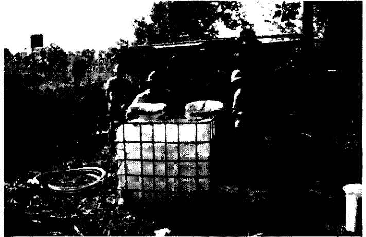
MW-13 mixing cement/bentonite grout
