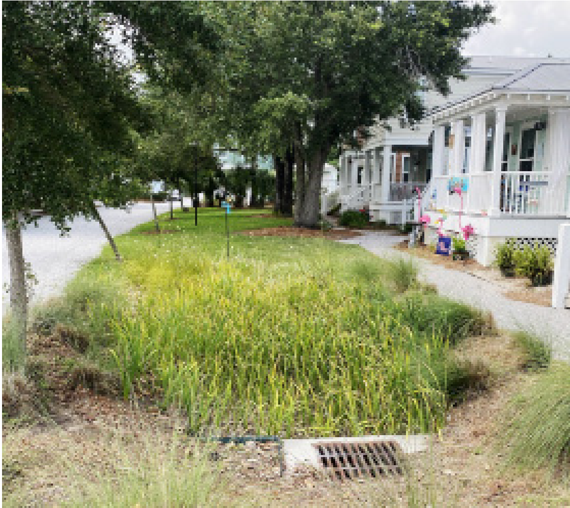
Figure 4-2. Residential rain garden at the Cottages at Oak Park in Ocean Springs, MS. (Photo: Kristen Sorrell, MDEQ)
