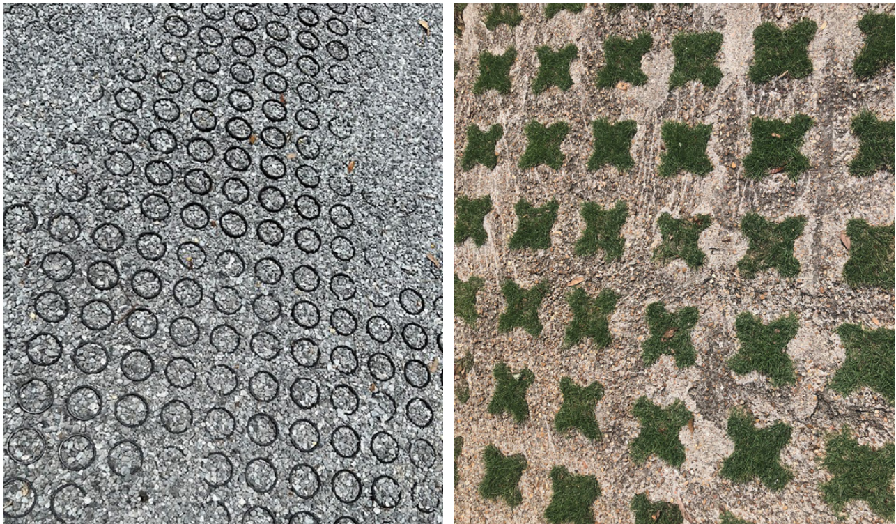
Figure 5-1. Close-up views of two types of permeable pavers. Openings filled with aggregate (left); openings filled with soil and planted with grass (right) (Photos: Kristen Sorrell, MDEQ).
