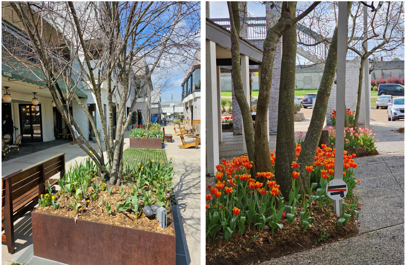
Figure 2-18. Disconnecting sidewalk runoff by redirecting flow into planter boxes is one strategy to manage stormwater flows in urban areas. (Photos: Natalie Segrest, MDEQ)
