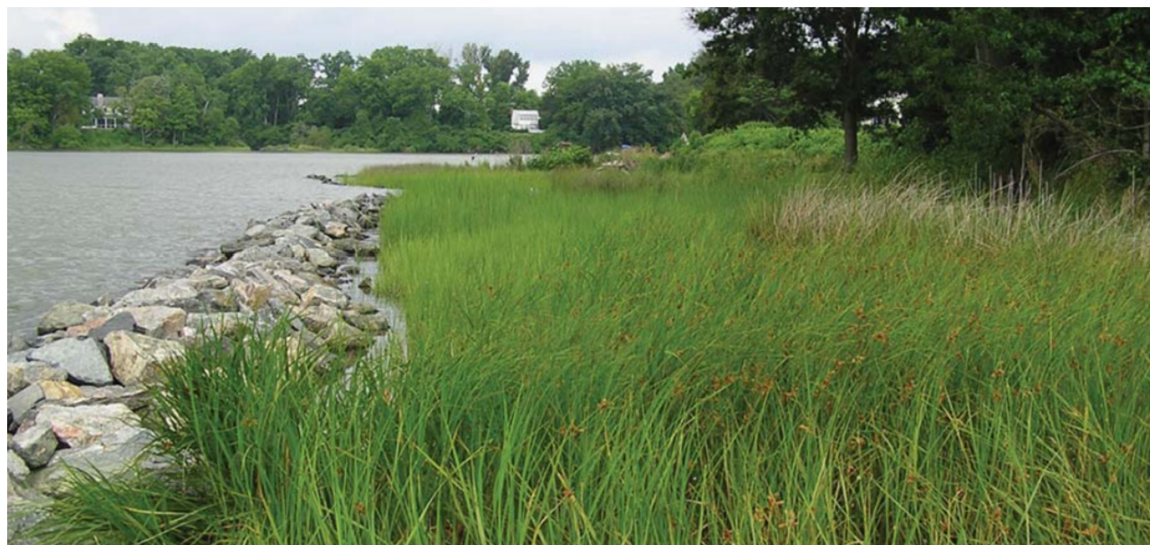
Figure 2-22. Rock sill with planted marsh, an example of hybrid design employing structural stabilization and living shoreline techniques. (Photo: K. Duhring, MDMR)
