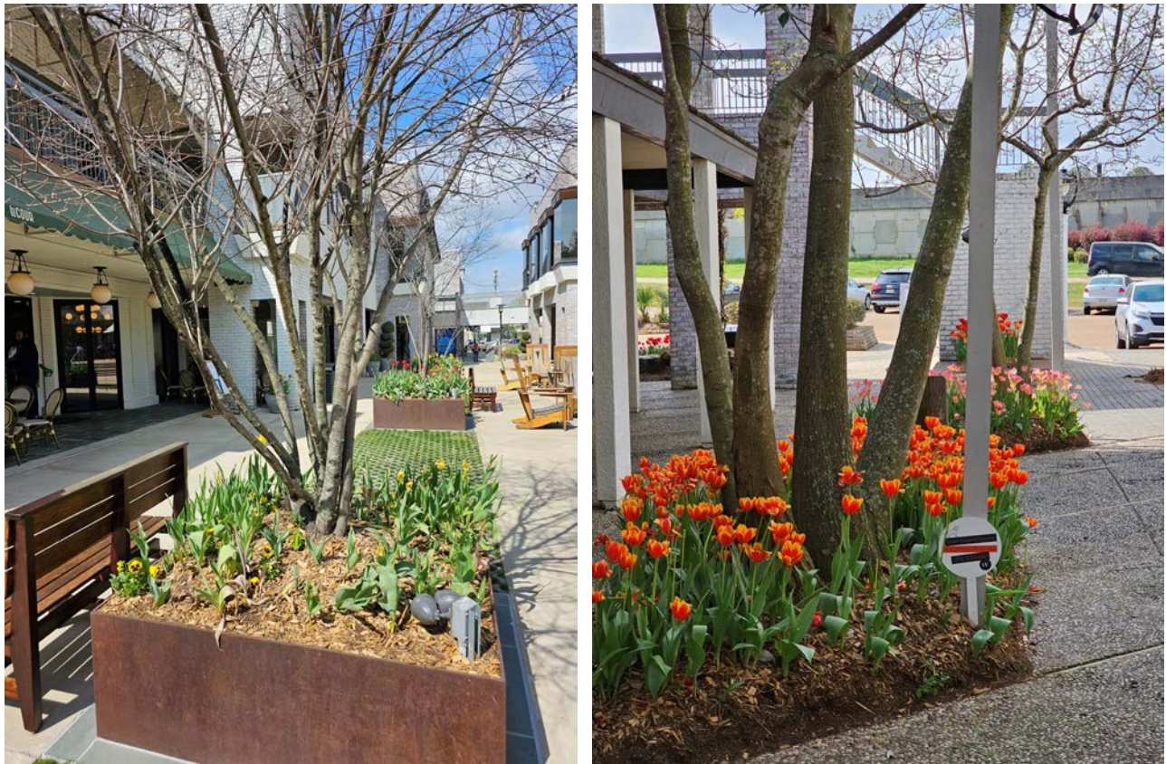
Figure 2-18. Disconnecting sidewalk runoff by redirecting flow into planter boxes is one strategy to manage stormwater flows in urban areas. (Photos: Natalie Segrest, MDEQ)
