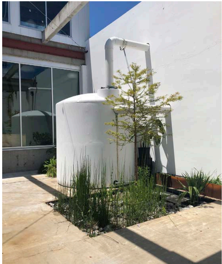
Figure 2-17. Rooftop downspouts directed to cistern and stormwater planter at Ecoshed in Jackson, Mississippi.
