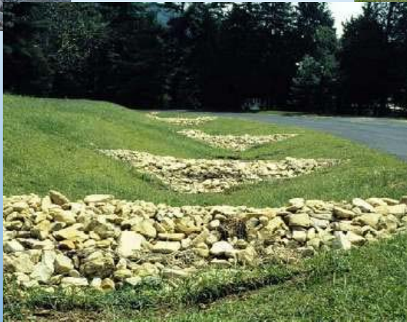
Grass Swale with Check Dams
