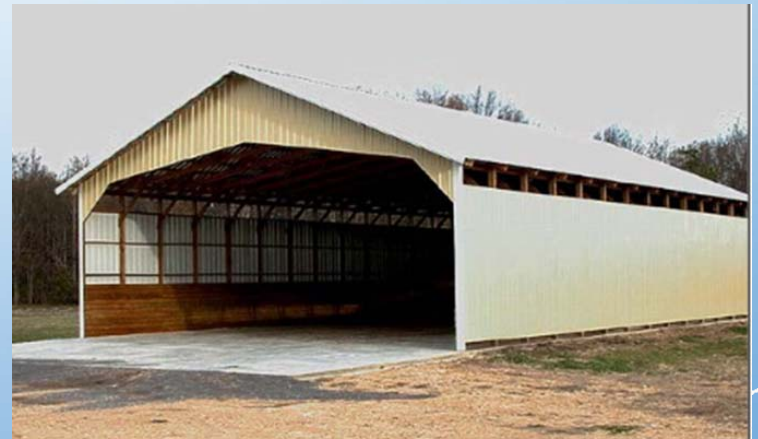
Dry Stack Building for Poultry Litter
