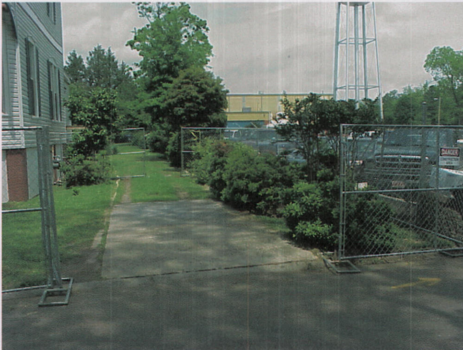
Photo 2 – The Frazier driveway prior to remedial activities. The temporary fence is shown in this view. This view is looking north from Lee Avenue.
