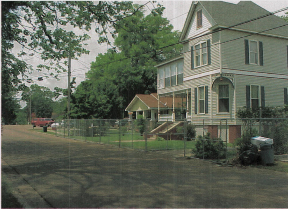
Photo 1 – View of the front of the Frazier property showing conditions prior to remediation activities. The fence is a temporary installation for public access control.
