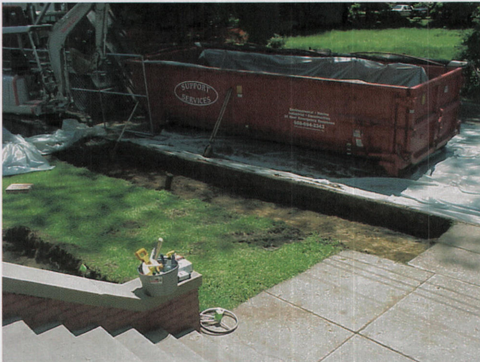
Photo 6 – View looking southeast showing completed excavation along Lee Avenue.
