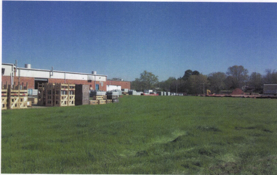
PHOTO 13 – View looking northwest of the final grass cover over the remediated area east of the plant building.
