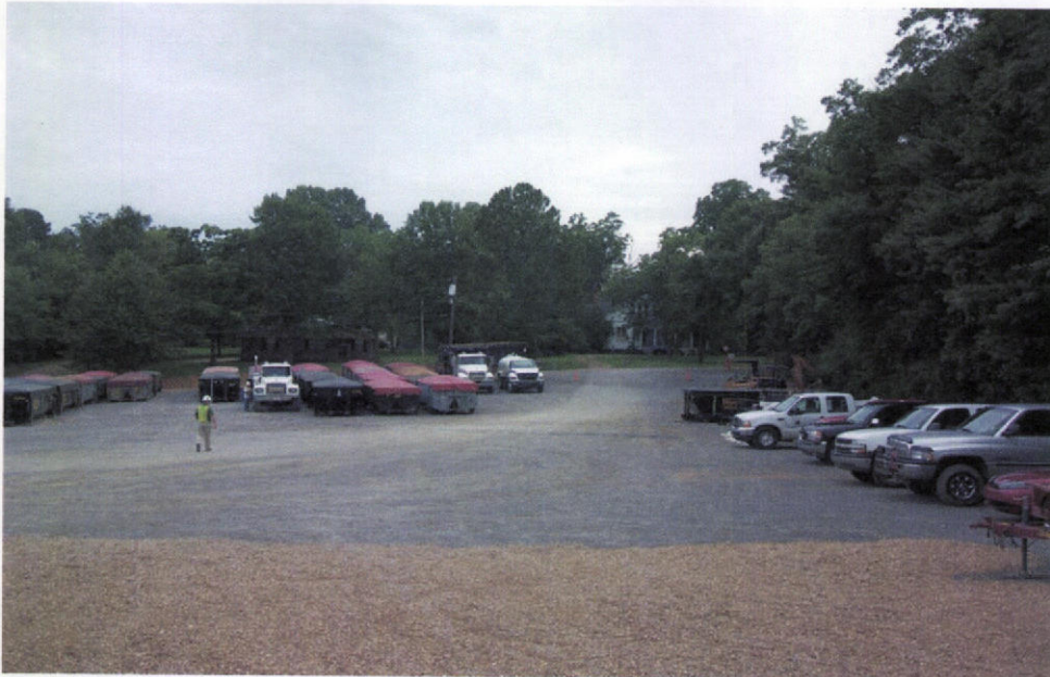
PHOTO 14 – View looking north of the remediated northeast quadrant of the property. The area is covered with gravel and is being used as the construction staging area for the offsite remediation work. Empty roll-off boxes are visible in the background.
