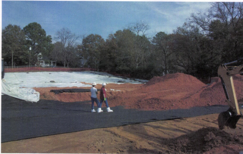
PHOTO 11 – Clean backfill is being placed over geotextile fabric in a remediated area in the northeast area of the plant site.
