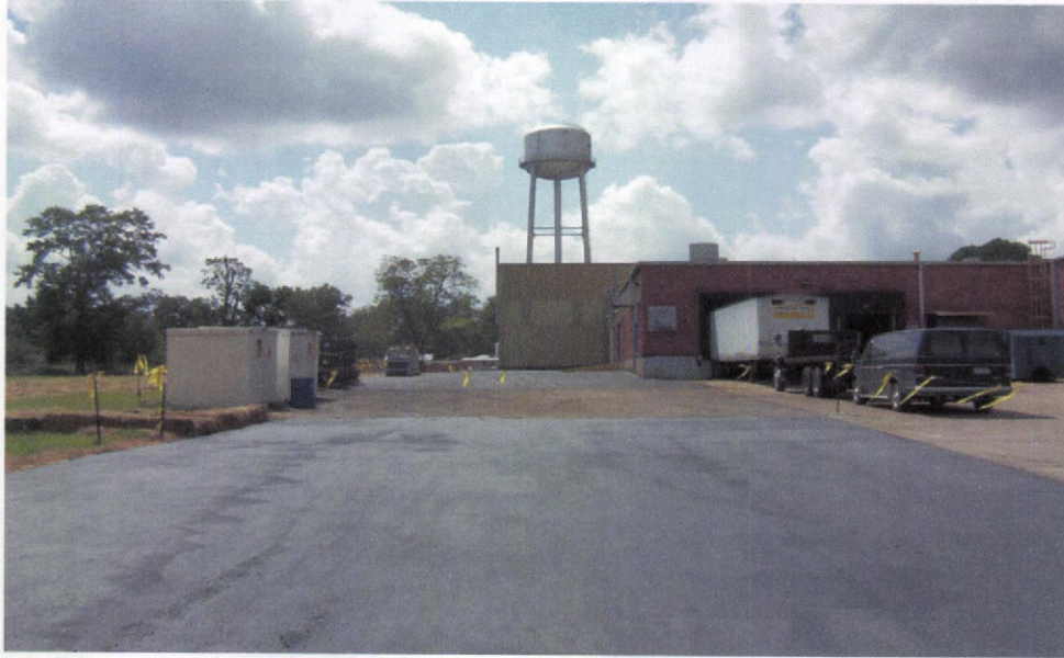
PHOTO 15 – View looking south along the east side of the plant building with asphalt cover in place over remediated areas.
